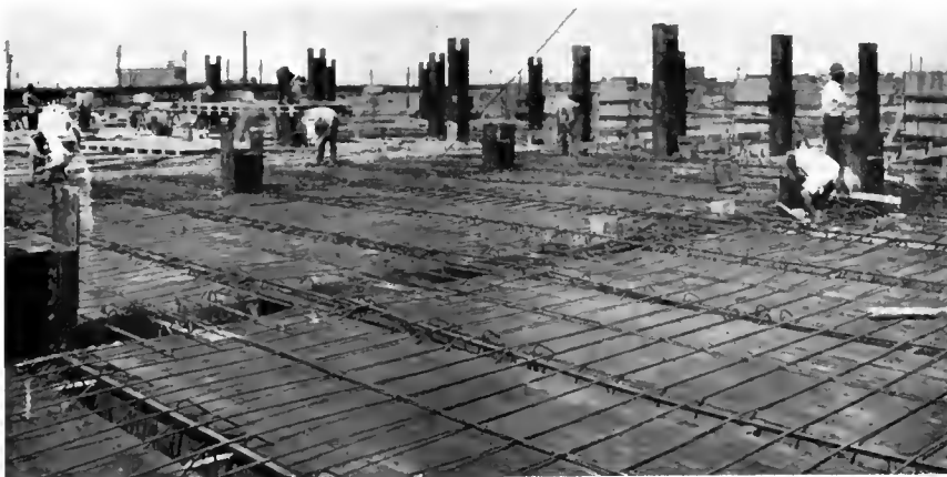
VIEW SHOWING SLAB REINFORCEMENT
